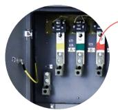
input terminals for connecting cables to the power supply
