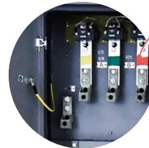
input terminals for connecting cables to the power supply
