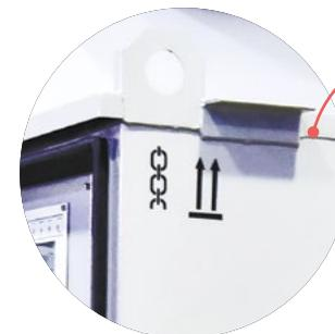
lifting lugs for loading and unloading the VSD
