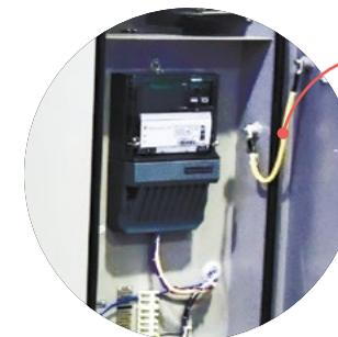
compartment for surface block and a compartment for an electric energy meter
