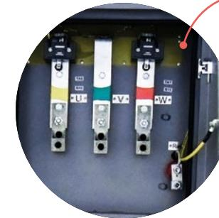
output terminals for connecting transformer and a terminal for combining a cable measuring motor+power cable insulation resistance
